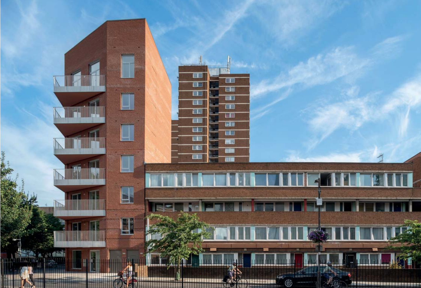
Marklake Court (formerly Kipling Estate Garages) / Bell Phillips Architects
